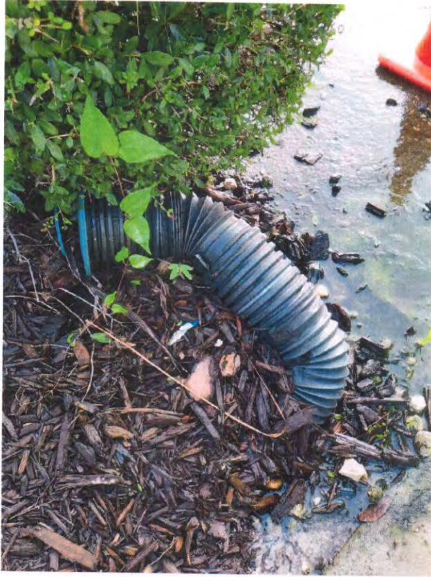
Damaged drain line (Before)
